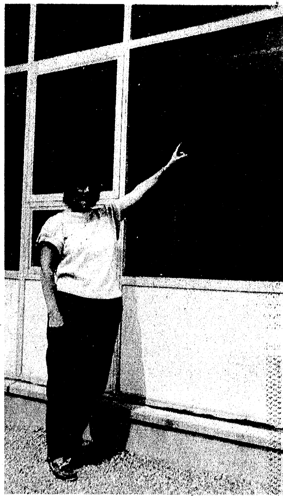
WINDOWS WERE BROKEN Sunday night at Beach and North schools by vandals who threw beer bottles at them. Sarah Joseph, a maintenance worker at North school, points to some of the damage.
